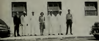
The plant and operating staff.
